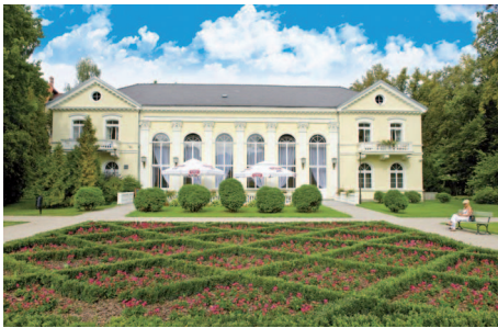
Picture 6. The Edward Pavilion
